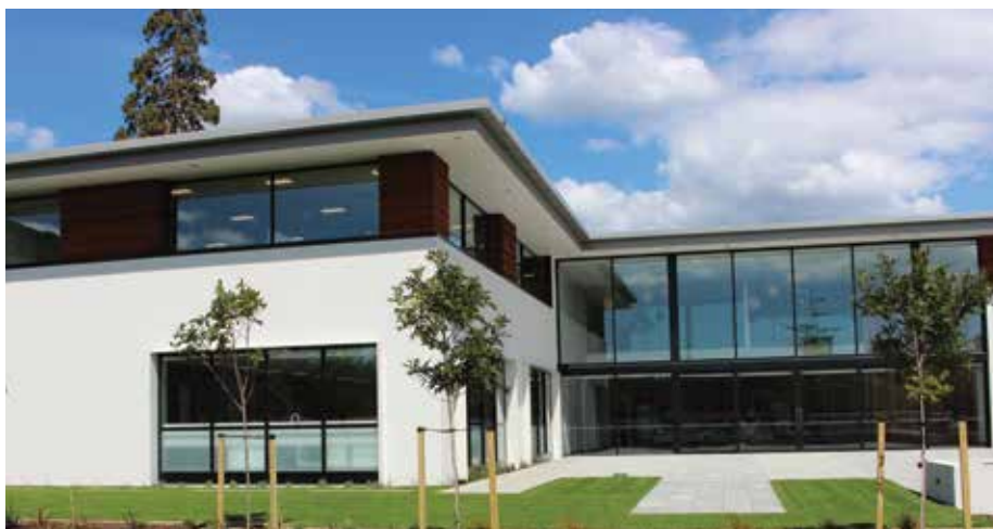
Exterior view of the new Cawthron Institute Envirotech Wing
