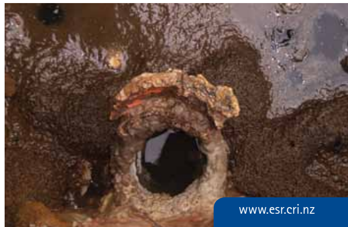
Below: Samples are taken from within the septic tank effluent pipe
