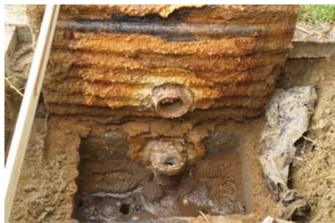
Open lid of septic tank – showing the effluent pipe
